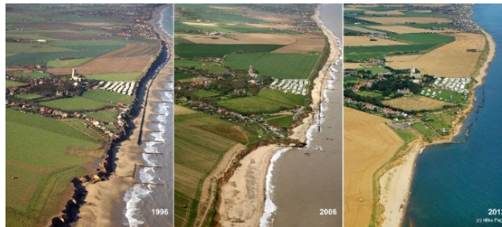
Happisburgh in 1996, 2006 and 2012 during which time it has lost a number of sea front properties Coastal Adaptation at Happisburgh (United Kingdom)
